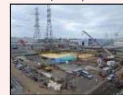
After dismantling in H1 east area
