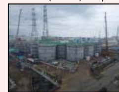
Start of dismantling in H1 east area
