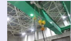
<Handling of the storage can lifting tool at the main hoisting>
