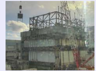
Dismantling of the windproof fences (as of December 19, 2020)
