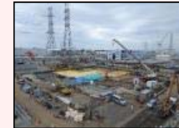
After dismantling in H1 east area
