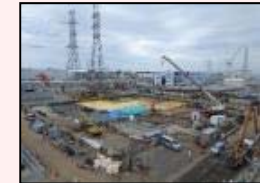
After dismantling in H1 east area
