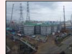
Start of dismantling in H1 east area
