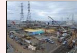
After dismantling in H1 east area
