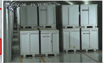
Solid waste storage facility
