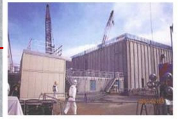
Temporary waste sludge storage
