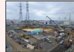
After dismantling in H1 east area
