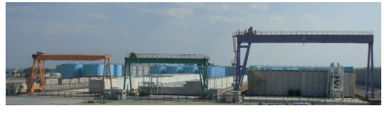
Spent adsorption vessel temporary storage facility
