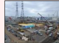
After dismantling in H1 east area
