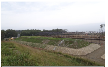
Temporary soil-covered type storage facility
