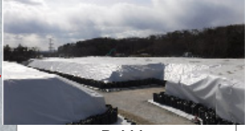
Rubble (outdoor accumulation)
