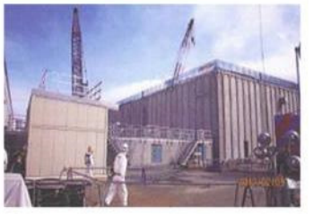
Temporary waste sludge storage
