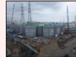
Start of dismantling in H1 east area
