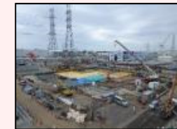
After dismantling in H1 east area
