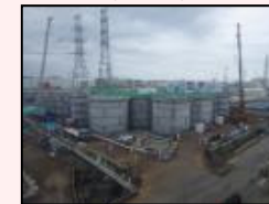
Start of dismantling in H1 east area
