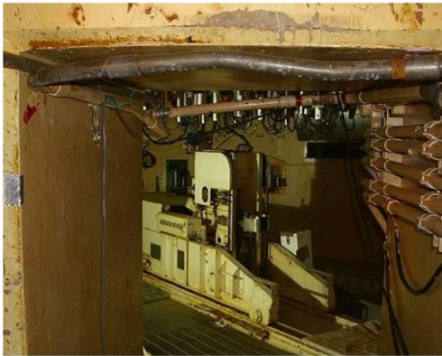
Looking inside through the pedestal opening
