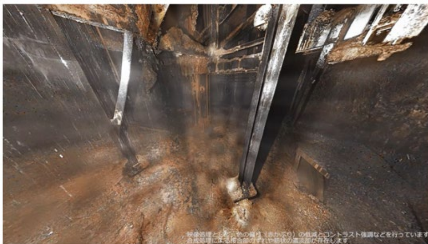
Figure 4.9.2-3 Images of the inside of the pedestal of Unit 2 (1/3) [2-21][2-22]
