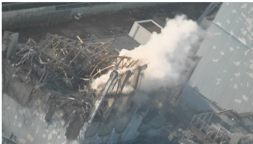
Figure 12 Aerial photo of Unit-3 (March 16 th , 2011)
