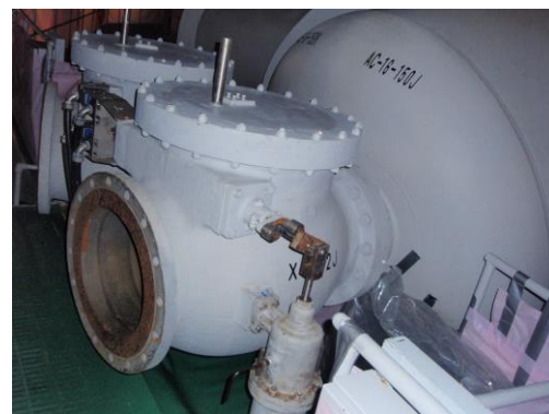
Figure 2 Vacuum breaker valve
