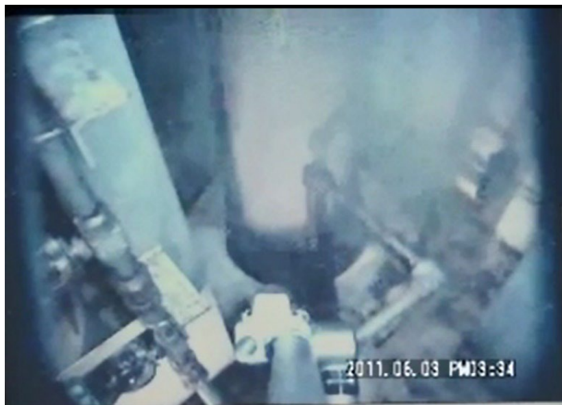
Figure 1.3 Steam observed at the southeast floor penetration of the 1st floor of Unit 1 R/B (June 2011) [3]
