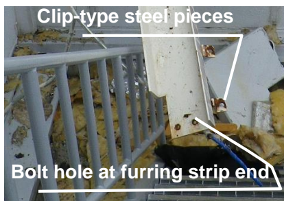
(B) Bolt hole at furring strip end
