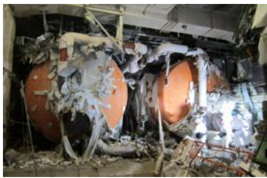
(A) IC tank south side (1)
