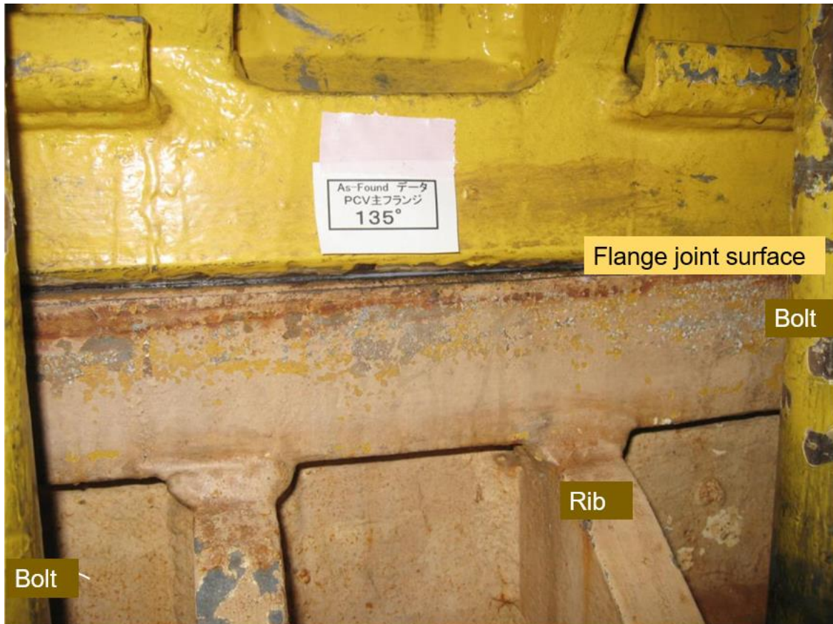
Figure 2-38 Flange of PCV lid before the accident [2-22]
