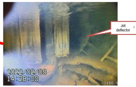
Status near east-northeast of PCV (overhead view)
