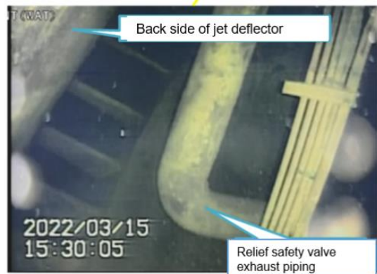
Photo 3. Status of jet deflector (G) back side
