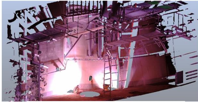
2nd floor shell wall east face (point cloud data)
