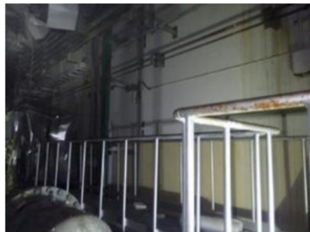
West face of pool wall on 4th floor (photograph)
