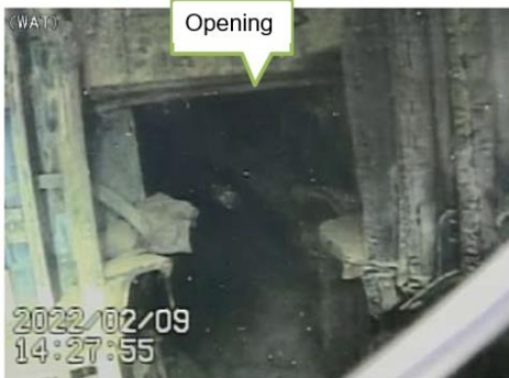
B. Overhead view of pedestal opening
