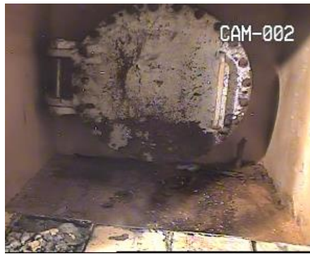
Flange of Penetration X-6 (after removal the iron plate)
