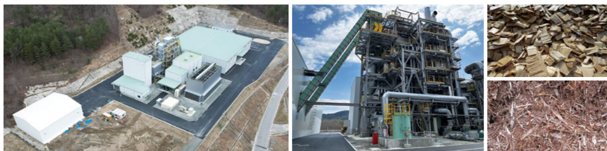
litate Mirai Power Plant
