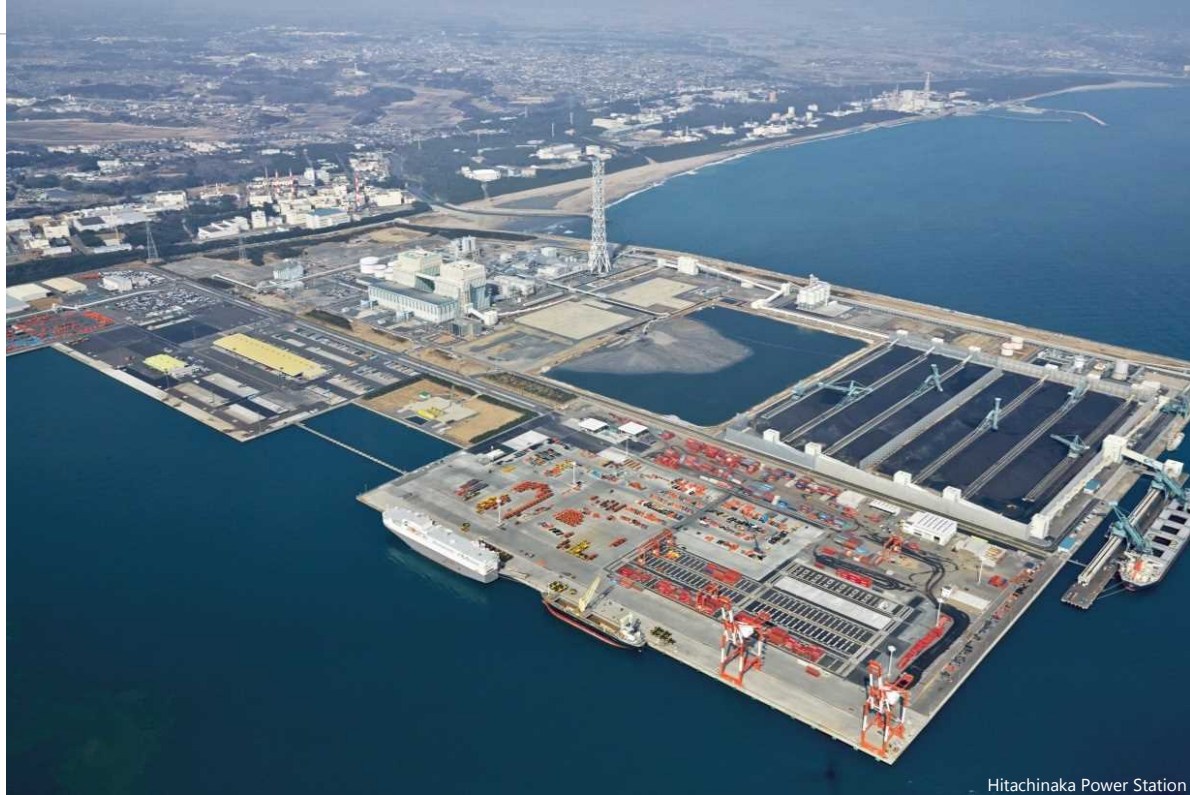
Hitachinaka Power Station
