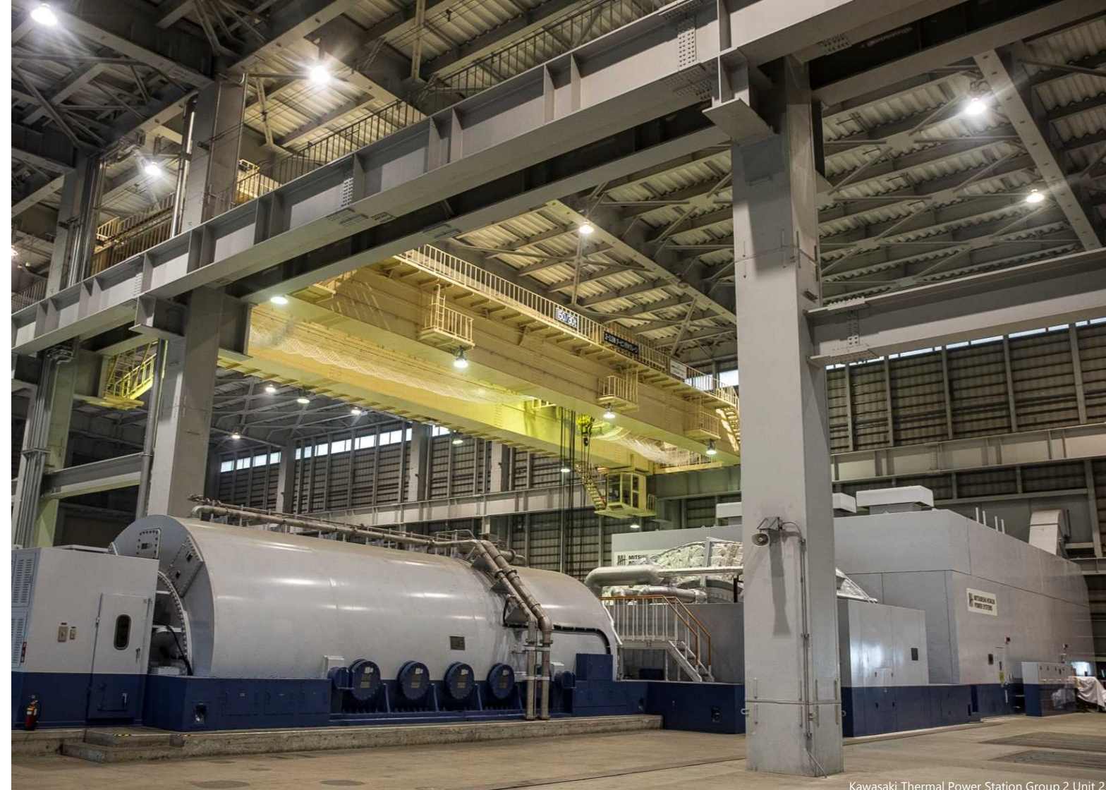
Kawasaki Thermal Power Station Group 2 Unit 2
