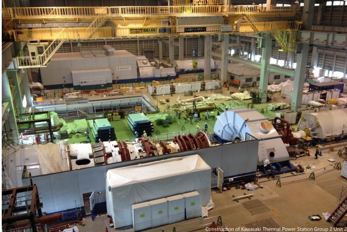
Construction of Kawasaki Thermal Power Station Group 2 Unit 2
