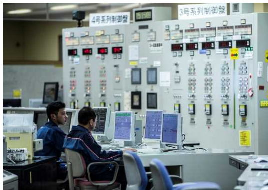
Central operation room of Futtsu Thermal Power Station
