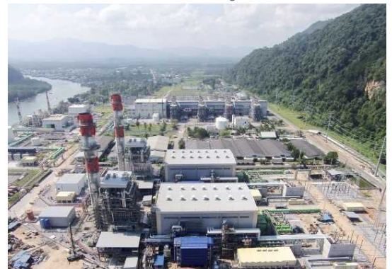
Khanom Power Station, Thailand
