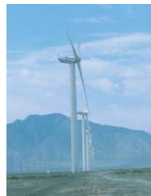
Wulabo Wind Power CDM Project in Xinjiang Uygur Autonomous Region, China
