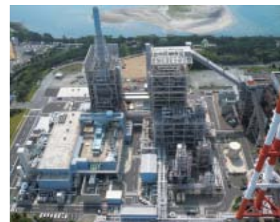
IGCC demonstration plant with power output of 250 thousand kW. Source: Clean Coal Power R&D Co., Ltd.
