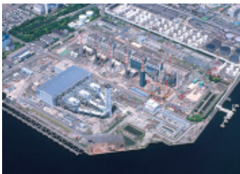
Kawasaki Thermal Power Station
