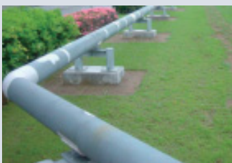
Switching to above-ground pipes
