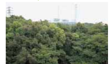
Sodegaura Thermal Power Station (photo taken in 2005, 21 years later)
