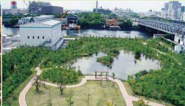
Biotope at the Shinagawa Thermal Power Station
