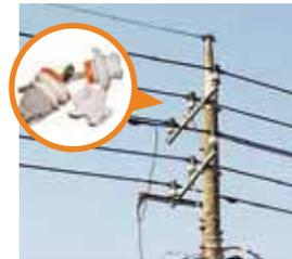
Attached to utility poles, insulators are made of ceramics that do not conduct electricity.
