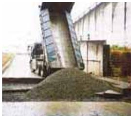
Concrete is used for roadbed material, iron reinforcement is recycled as raw material for steel.
