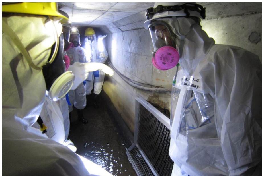
FIG. A-3. Inside K drainage channel during the site visit
