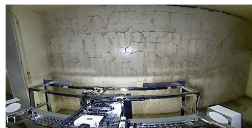
②高所壁面除染前
