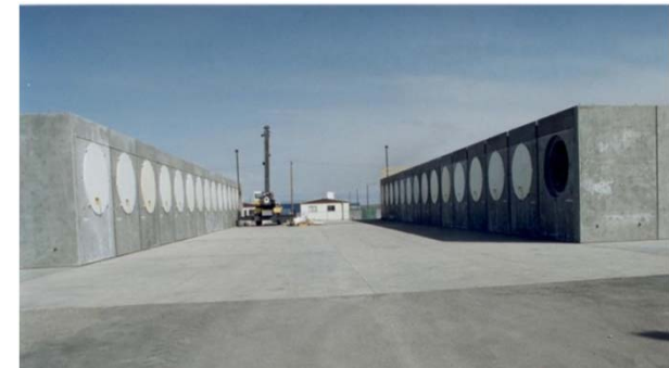
米TMI-2燃料デブリの保管システム(参考) 出展:Andrew P. Szilagyi, Three Mile Island Unit 2 Overview and Management Issues, OECD-Nuclear Energy Agency – 12th Meeting of the WPDD, France(2011i)より
